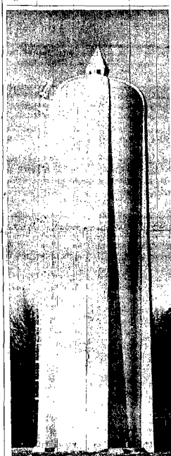
WAYNE'S NEW WATER tower will be the same as this one. Capacity will be 750,000 gallons and, used along with the present tower, will give Wayne more water pressure and also a greater emergency safety factor.
